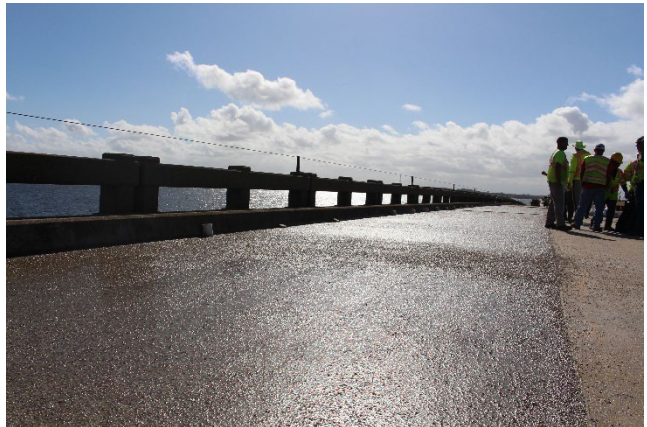
WLV+ seal coat layer
