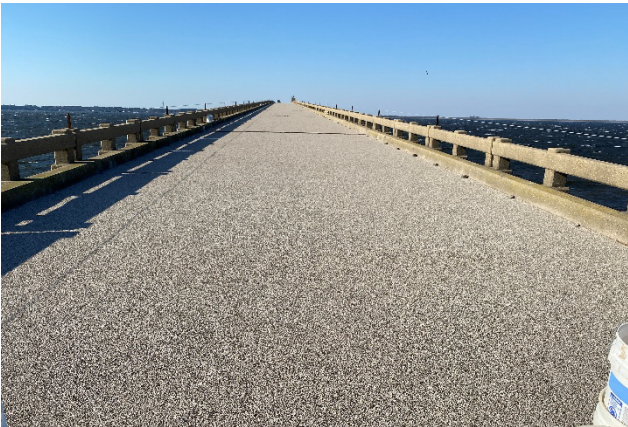
WLV+ Layer with aggregate
