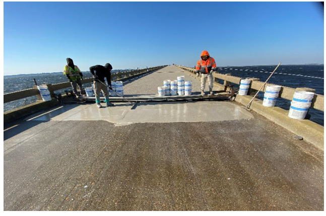
Matacryn WLV+ slurry wear coat application
