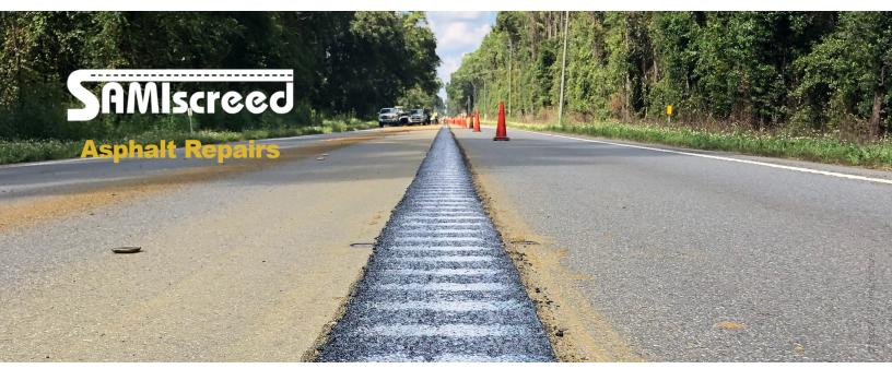
SAMIscreed is a hot-applied, flexible repair mastic for asphalt pavement defects. It is a highly-modified asphalt binder that is premixed with small aggregate, graded filler, steel fibers and recycled tire rubber. The factory-blended mixture provides more structural integrity than traditional hot-pour crack sealers.
